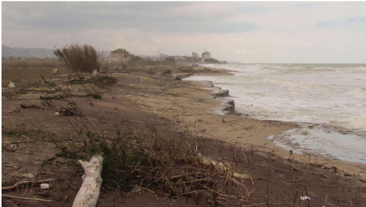
Fig. 2. Erosion caused by an eastern strong storm in 2013. Note the presence of mini-cliff and scour on the shoreline and reddish garnet sand on the backshore due to selective sorting by the backwash.
