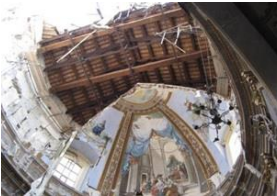
Figure 22. Collapse of the roof and of the decorated thin vault of St. Maria in Via Church [9].
