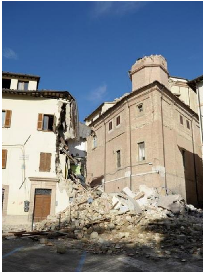
Figure 21. Collapse of the bell-tower of St. Maria in Via Church [9].
