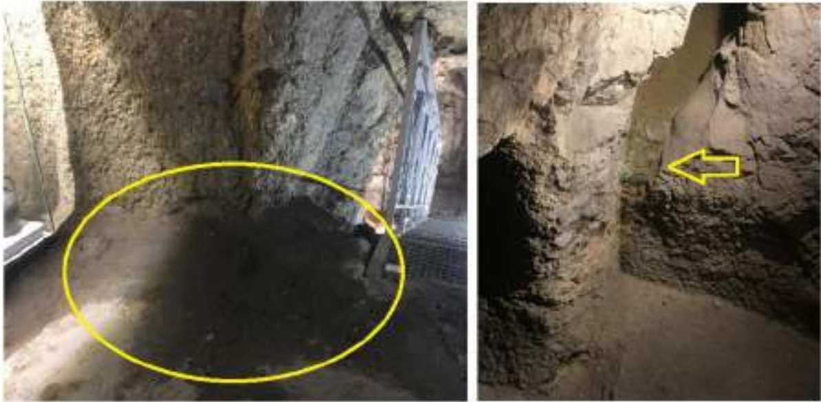
Figure 2.23. Traces of moisture inside the caves in the upper castle (left), impact of the additional moisture can be seen on the remaining tertiary sands inside the cave (right), as green algae. Photo: E. Streberová.
