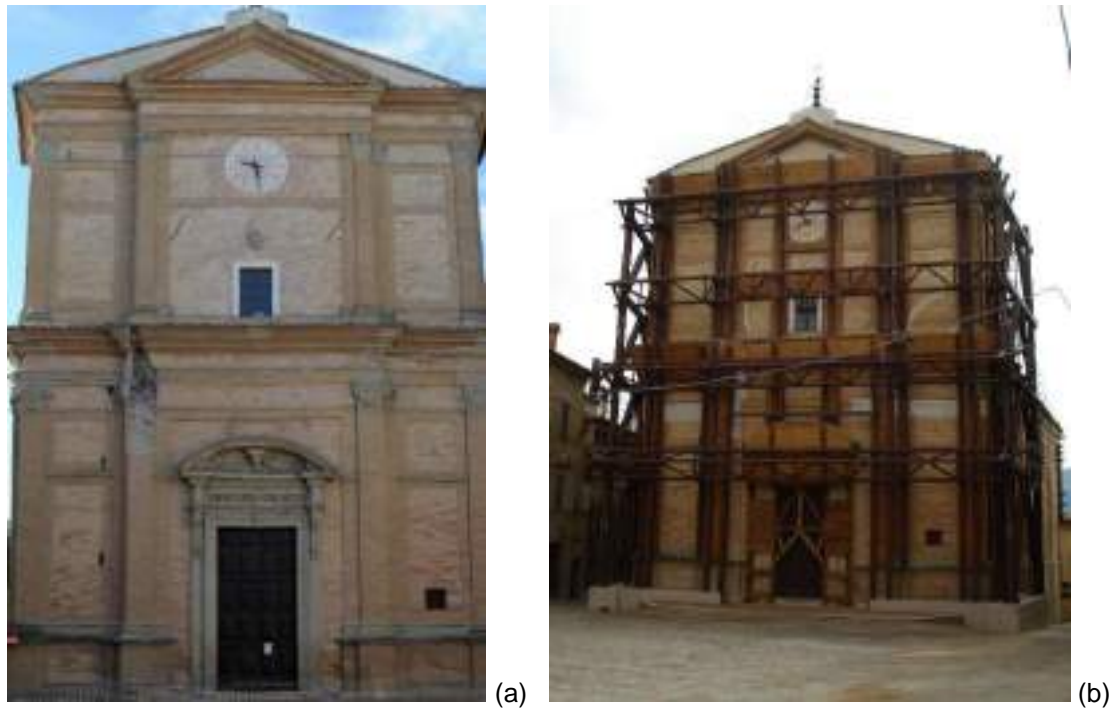
Figure 20. (a) Facade of St. Maria in Via Church and (b) the provisional steel structures that were put up in order to reinforce the remaining structures [9].
