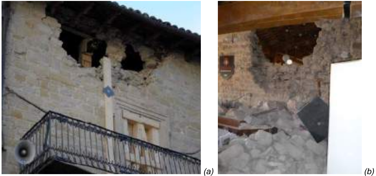
Figure 19. External (a) and internal (b) damage to and collapse of masonry (Ducal Palace) [9].
