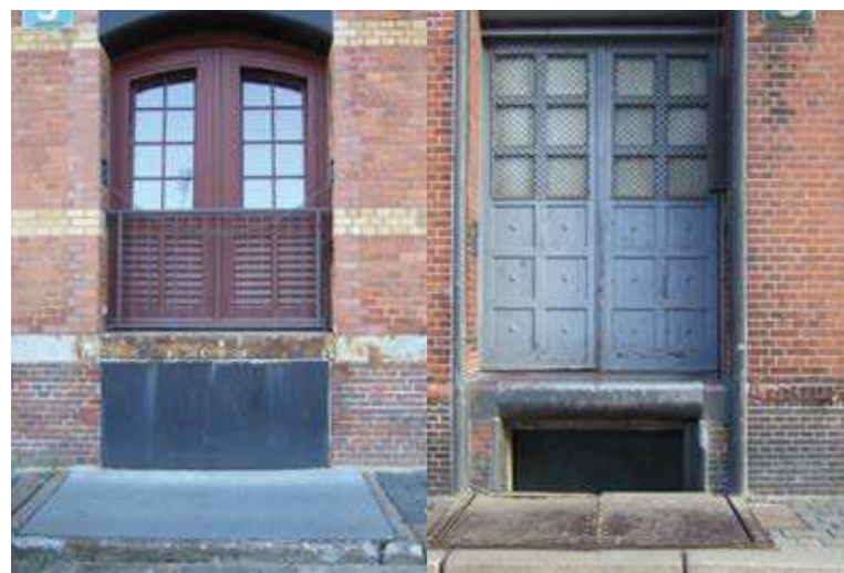
Figure 30: Sealing of a basement hatch with concrete
