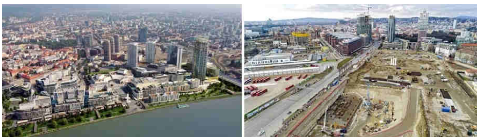
Fig. 10 New development of Downtown and new bus station under construction. Sources: https://www.autobusovastanica.sk , www.bratislavskenoviny.sk
